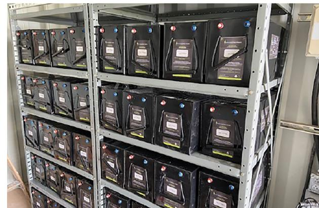
*Like other stationary storage battery platforms, UEP’s technology offers the advantages of modularity—but  $ZnMnO_2$  batteries also are based on materials that are globally abundant and not subject to thermal runaway.*
